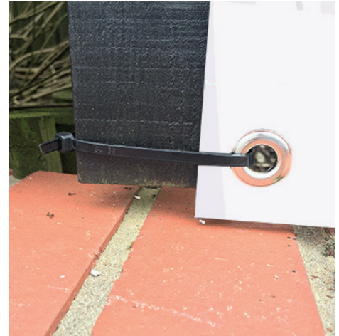
Fixings should be pulled tight
